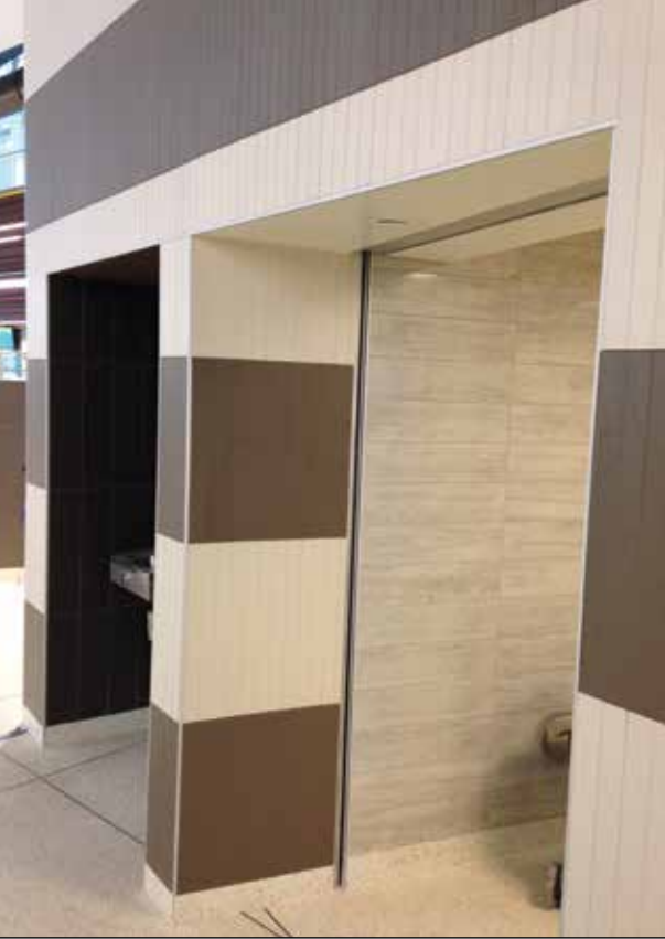
Entryway to bathrooms in progress
