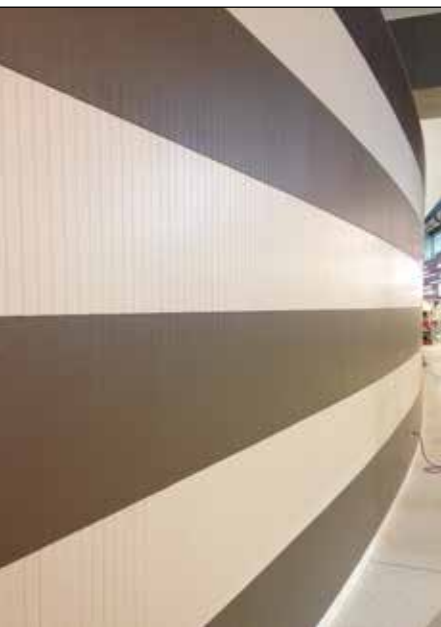
Tile wall in main terminal
