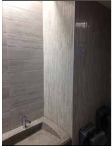
Finished tile in the bathroom sink area
